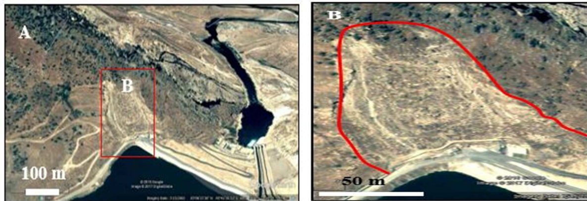
Figure 6: A) Google Earth image shows unstable slopes along the left bank of upstream slopes ( Station 1 ). B) Details of the main landslide. The red line represents the main unstable slope
