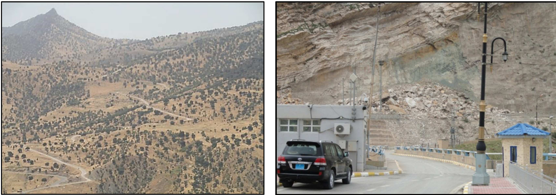
Figure 12: Upstream slopes of the Darbendikhan Dam. Left) Constructed unpaved roads with haphazard road cuts, Right) A rock fall in the day light slopes of the Pila Spi Formation.
