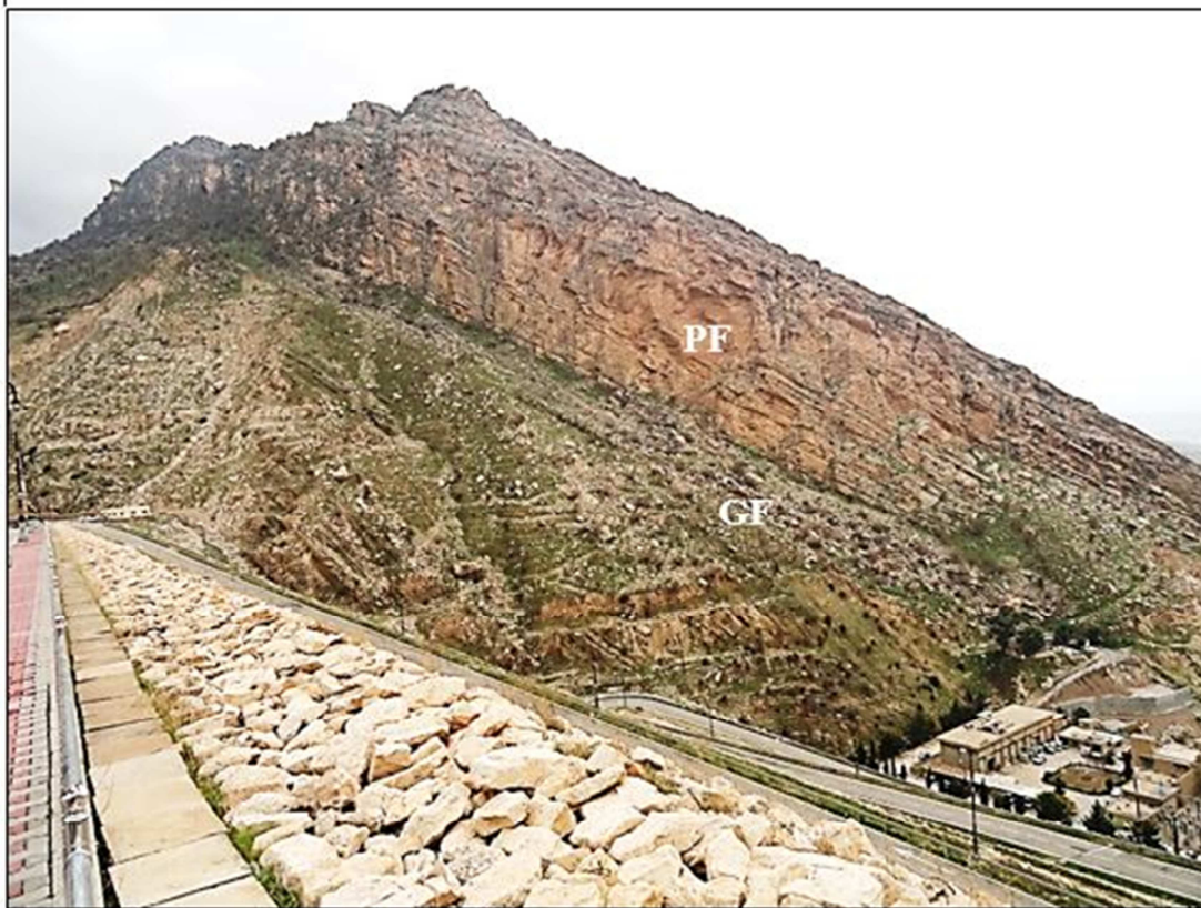
Figure 5: The crest of the Darbendikhan Dam, in the back ground is the Gercus Formation ( GF ) overlain by the Pila Spi Formation ( PF ). Note the fallen rock blocks from the Pila Spi Formation and the unstable slopes within the Gercus Formation.
